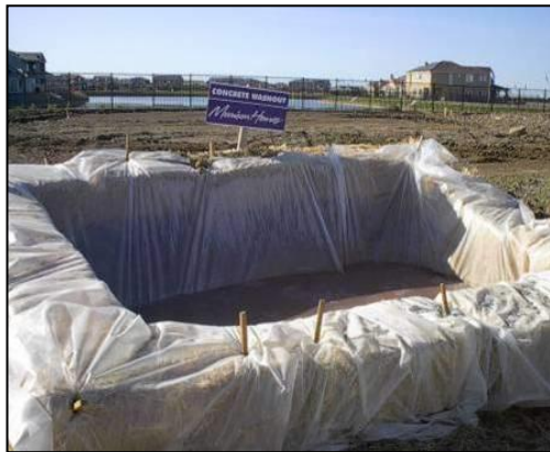
Plate 3-1 Typical concrete wash out areas
