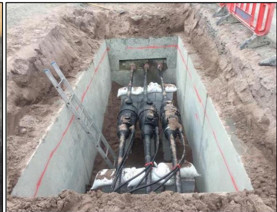
Plate 2-5 Joint Bay with Cable Jointing
